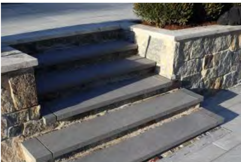
Mitered steps and custom drains
